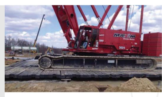
Struxure™ SR (steel reinforced) heavy-duty mats, made from structural polymer composites (SPC), when combined with A36 reinforced steel 1/4" or 1/2" steel flitch plates and MatLok™ hardware systems are more rigid, allowing them to be able to support more load than traditional 12" hardwood lumber mats for use under heavy equipment in wet or challenging project site conditions.
