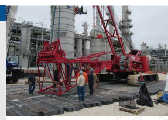
Struxure<sup>™</sup> Composite Construction Mats are engineered using a patented Recycled Structural Composite (RSC) formula—making them extremely strong, durable and impervious to rot, fungus, insects, and moisture.
